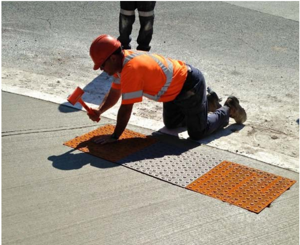
Photo - Public Works employee installing a tactile attention indicator.
